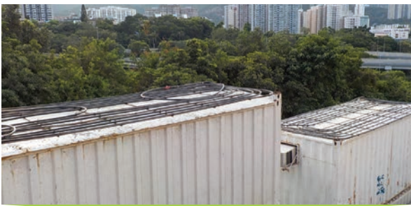
A 200m-long plastic hose arranged on the roofs of two site containers provided a solar hot water supply to a portable shower room on our foundations project in To Shek. On a sunny day, enough hot water is produced for five consecutive showers.
